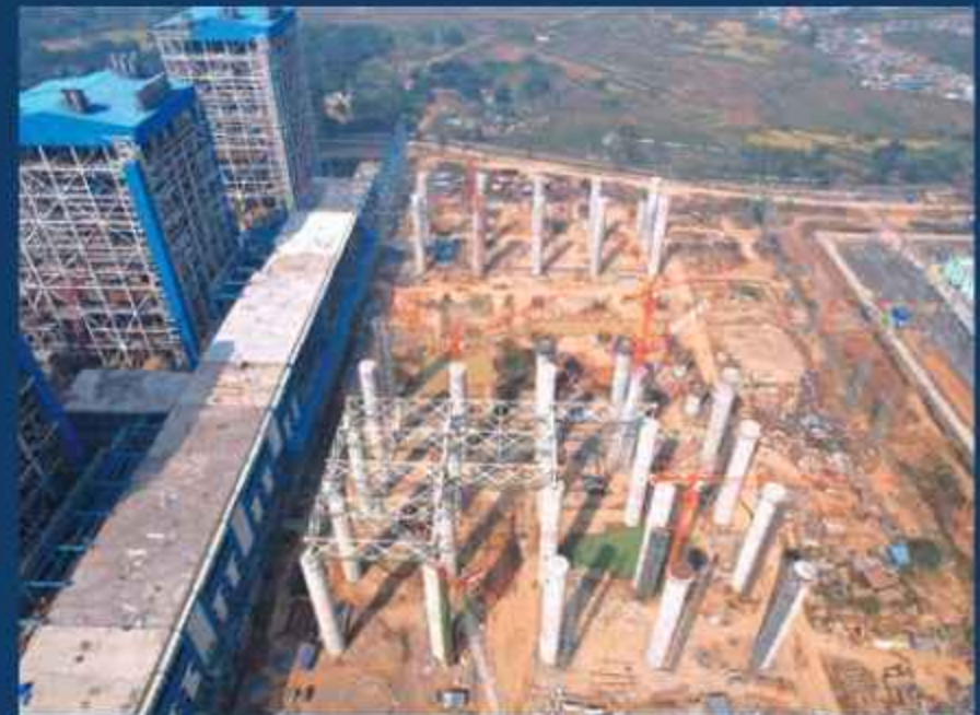
Air Cooled Condenser (ACC) under implementation at NTPC Patratu
