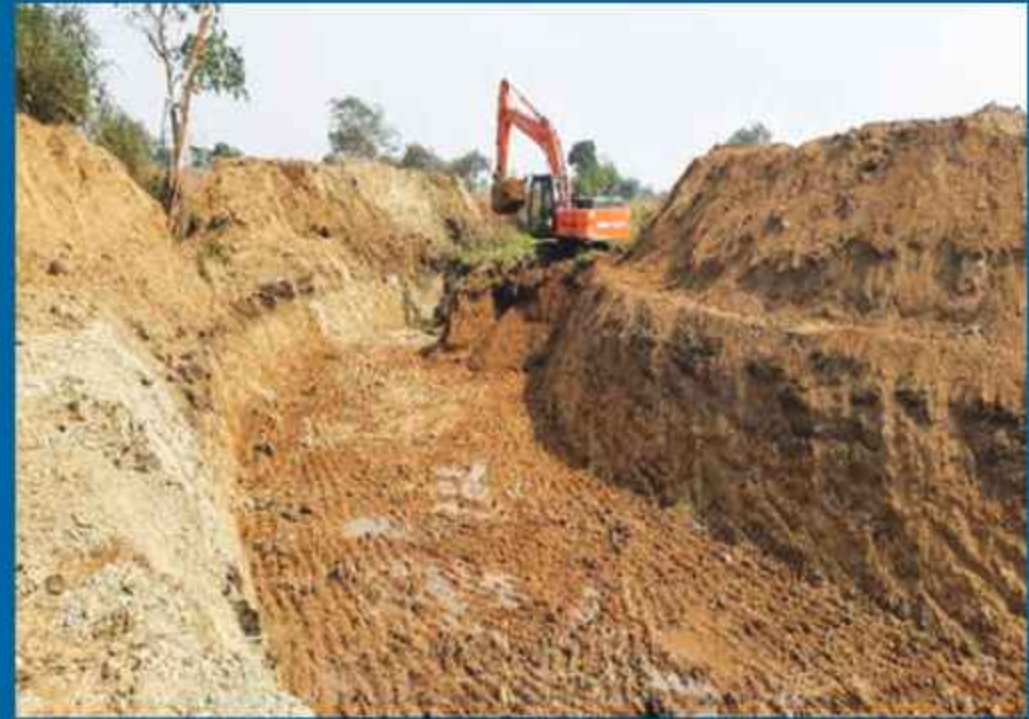
Deepening of nullah by machine operator Location- Sawergaon
