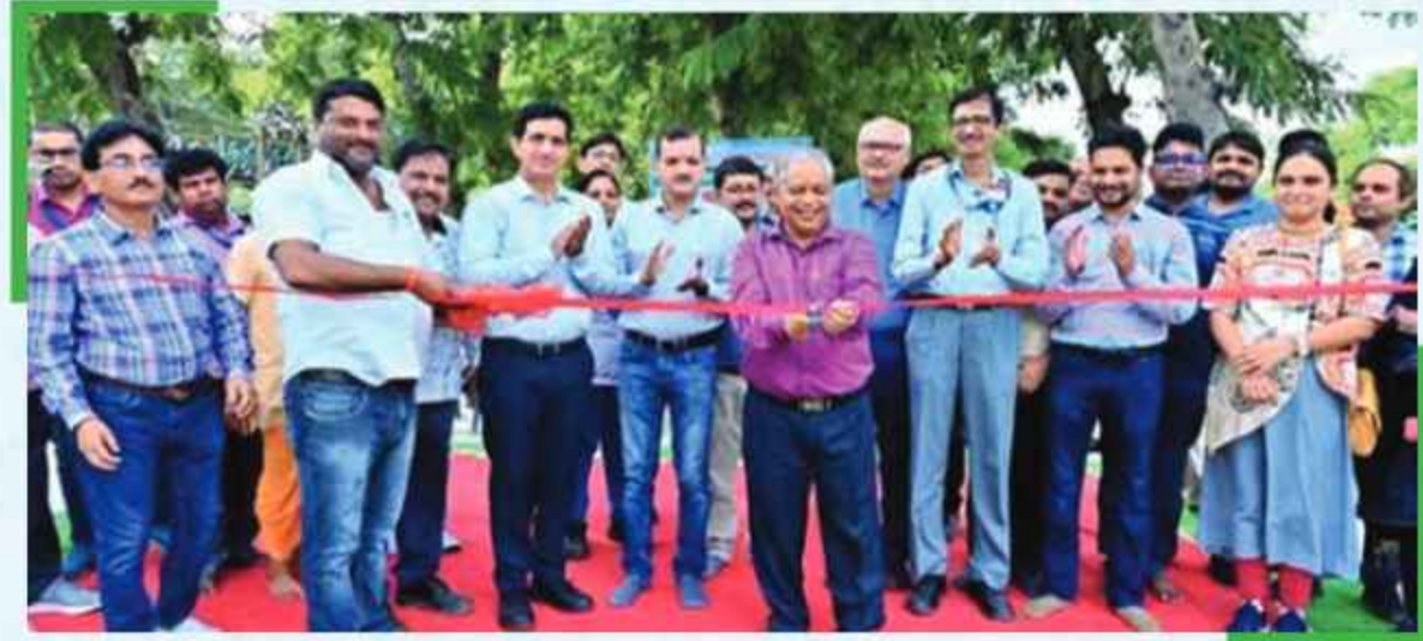
Drip irrigation in township horticulture for reuse of treated STP water at NTPC Tanda. The scheme was inaugurated by CGM Tanda on 29.08.2023
