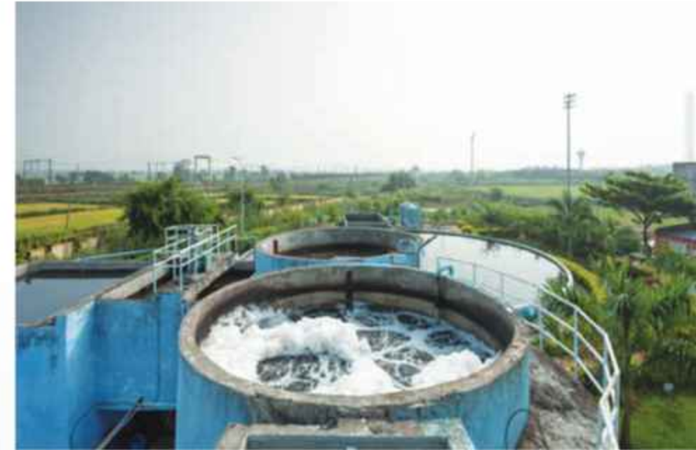
Sewage Treatment Plant
