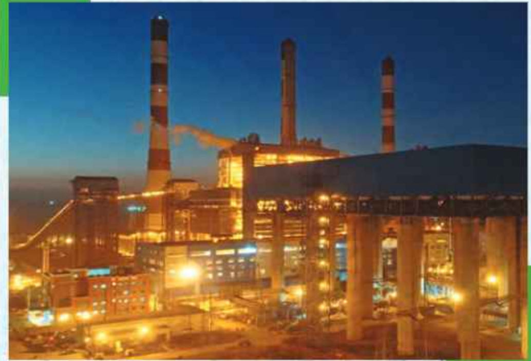
Air Cooled- Condenser at NTPC Patratu
