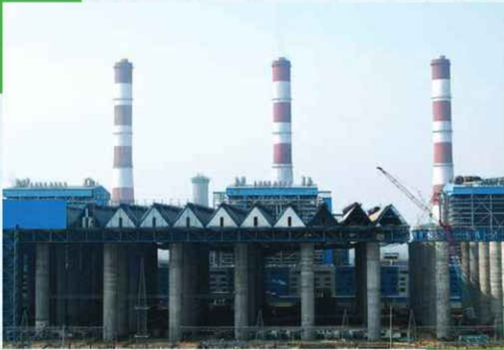
Air Cooled- Condenser at NTPC North- Karanpura
