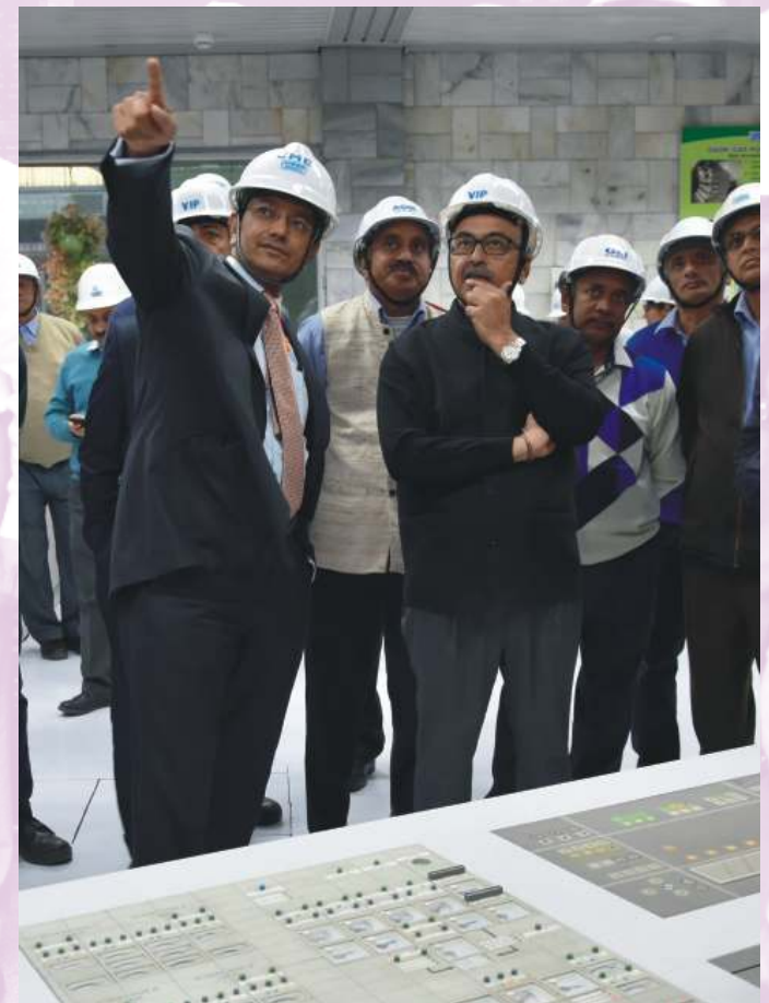
Shri A.K. Bhalla, Secy. (Power), GoI at NTPC Dadri Control Room
