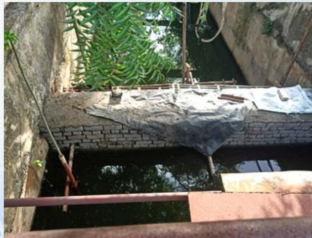
Use of Storm Water Channel as Rain Water Storage Facility
