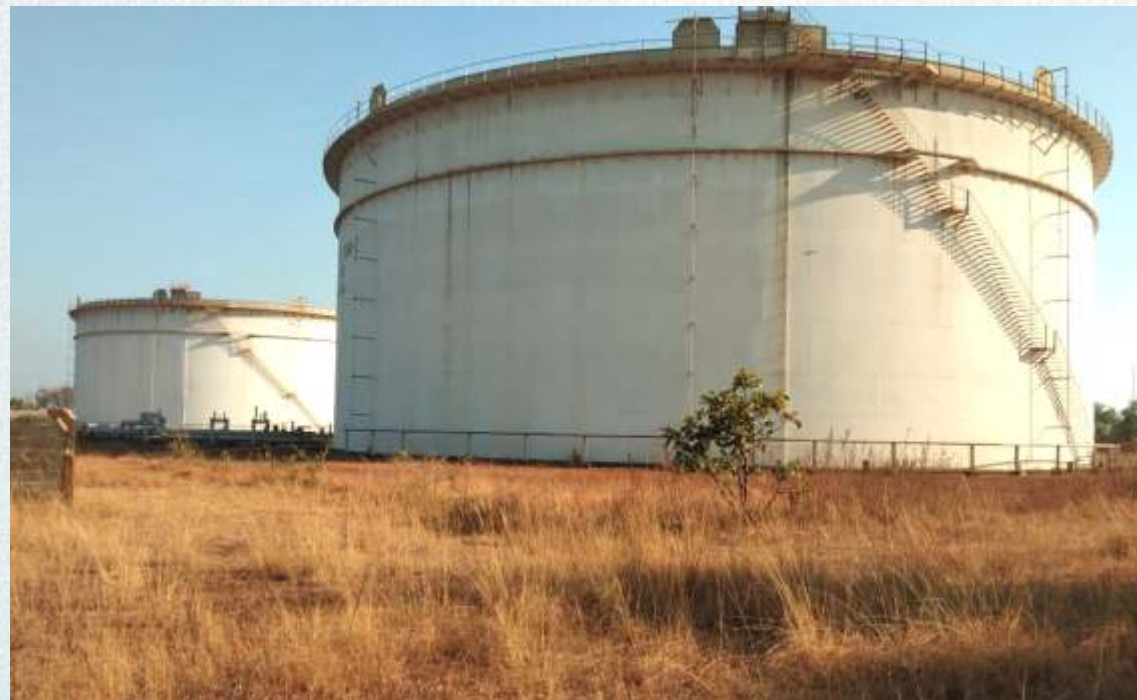
Storage tanks with total capacity of 1.6 Lakh M 3
