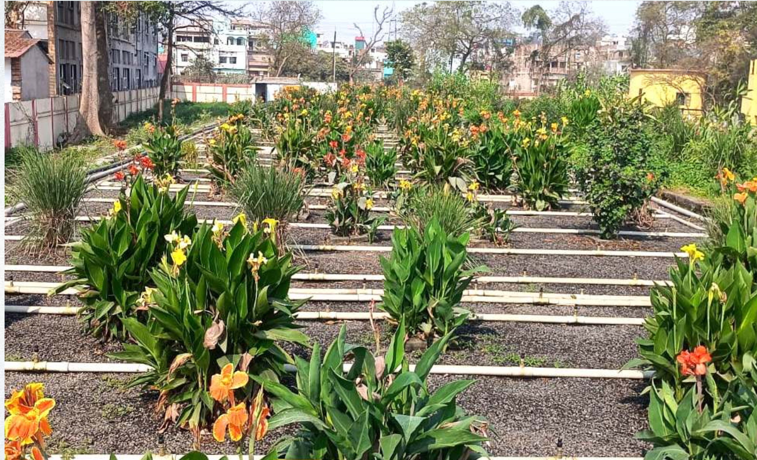
SBT Bioreactor-1 of NTPC Kahalgaon
