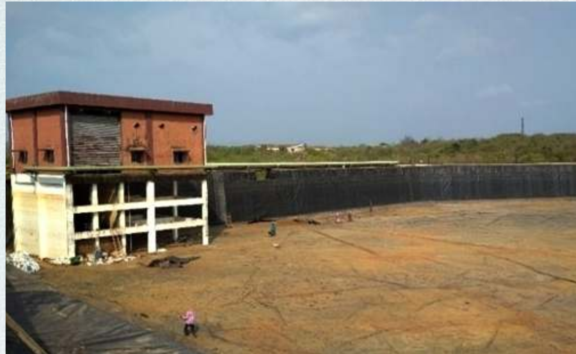
Lining of Water Reservoir of 1.2 Lakh m 3
