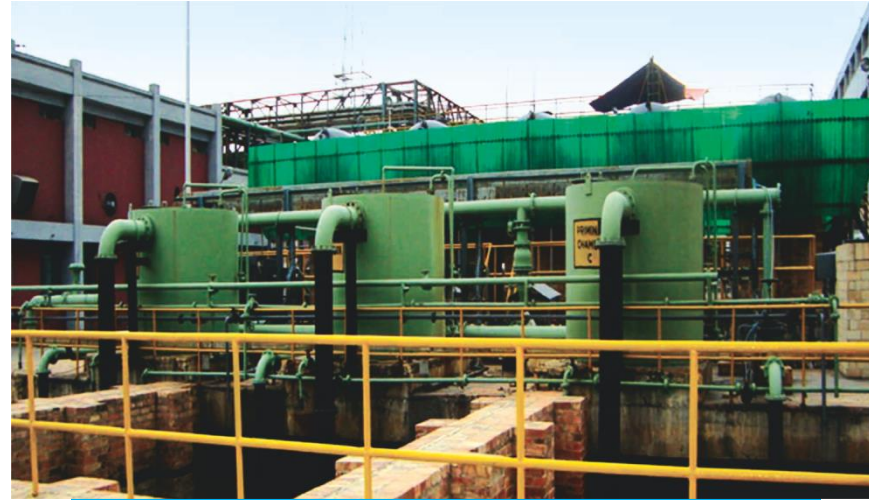
Neutralization Pit at DM Plant
