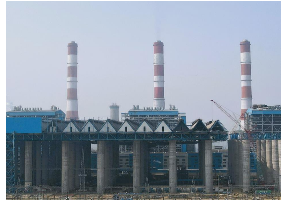
Air Cooled- Condenser at North- Karanpura
