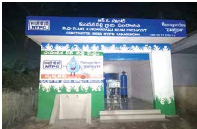
RO-Plant in Kundanpalli GP (Ramagundam)
