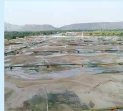
Reuse of water for Dust Suppression in Ash pond
