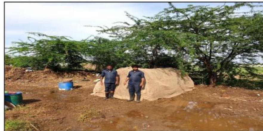
Cover with Jute cloth and maintain in moisture condition for 45 days
