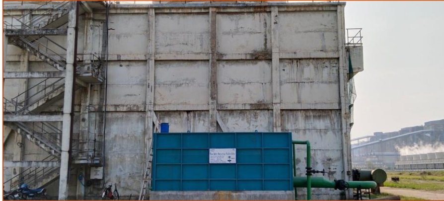
RWH Structure near Cooling Tower 1B
