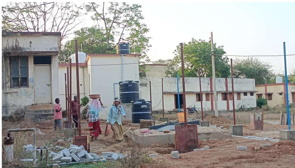
Fig 1 – Rain Water Harvesting in progress at Sipat Primary Health Centre
