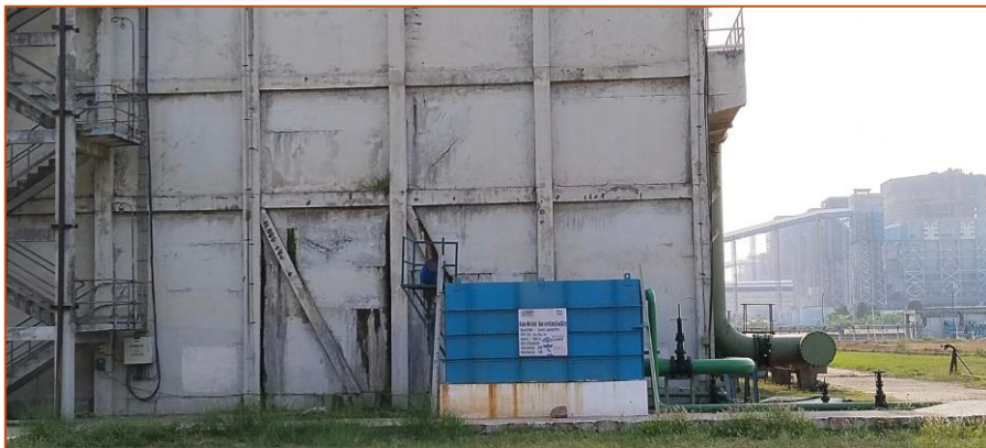
RWH Structure near Cooling Tower 2B
