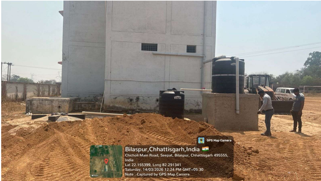
Fig 2 – Rain Water Harvesting in progress in Swami Atmanand school
