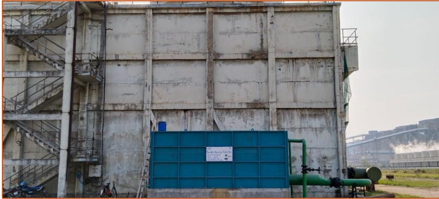
RWH Structure near Cooling Tower 1B
