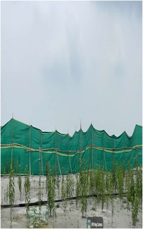
Shade net/Agro mesh Installation.
