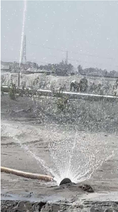
Installation of Water curtain.
