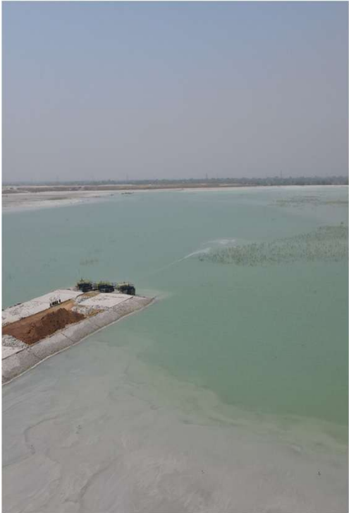
Ponding of charged Ash dyke
