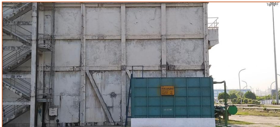
RWH Structure near Cooling Tower 3B
