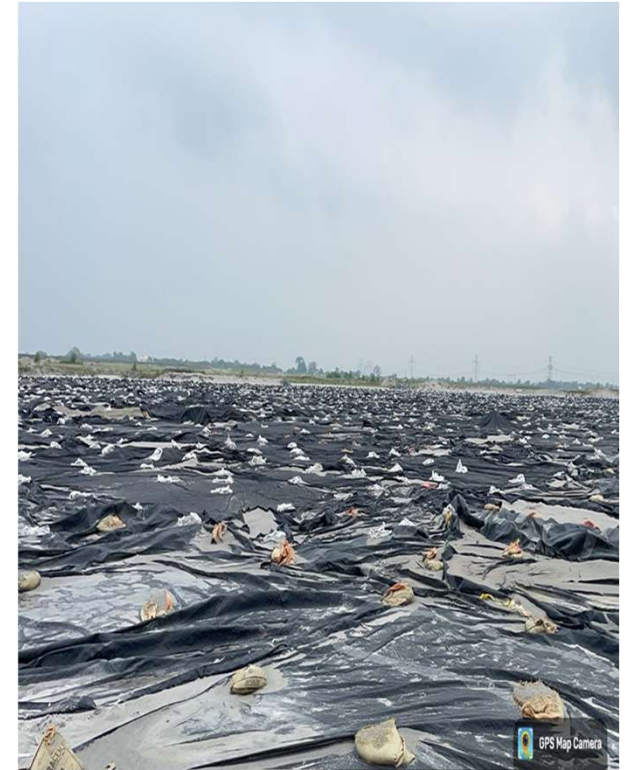
Laying of Tarpaulin Sheet.
