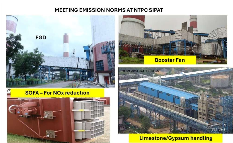
Fig 4: Emission Control technologies – DeNOx and FGD
