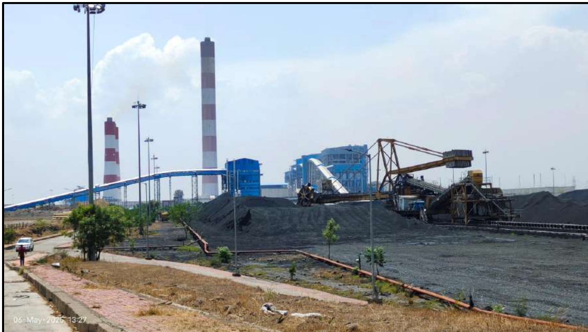
Figure 1: Landscape View of Khargone Super Thermal Power Station (KHSTPS).
