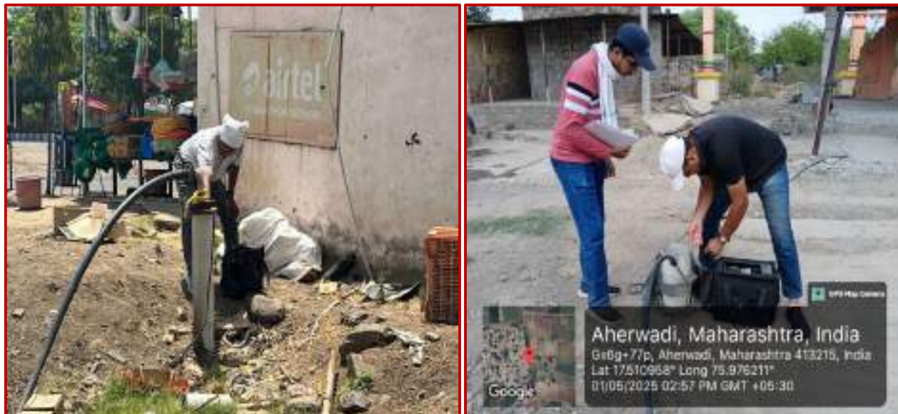
Plate 22-23 : Bore wells in the study area
