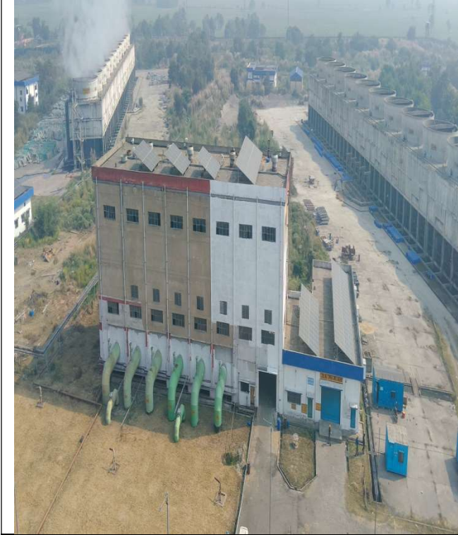
Roof top solar systems at CW Pump House
