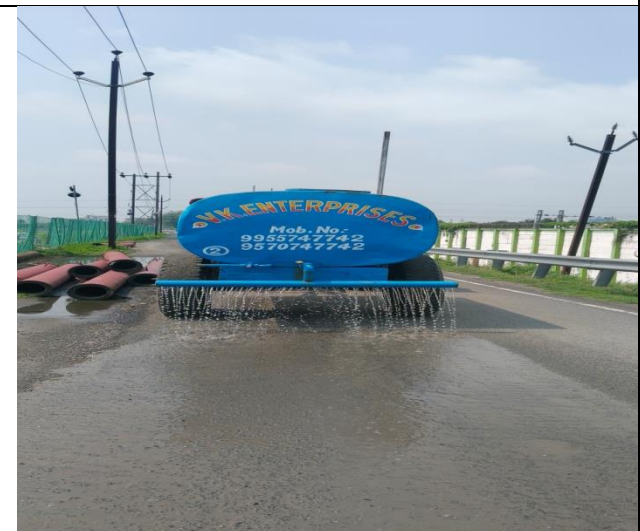
Water Sprinkling at road along Ash dyke boundary
