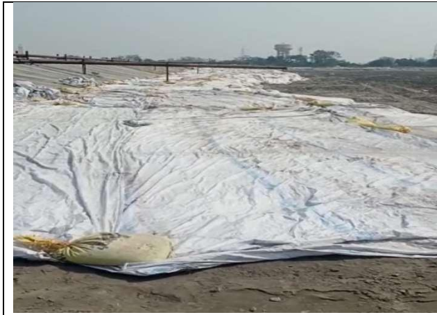
Covering of Dry patches with Waste Tarpaulin Cover at L1 Ash Pond
