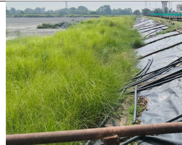
Green grass at Bottom of Slope of Ash Ponds
