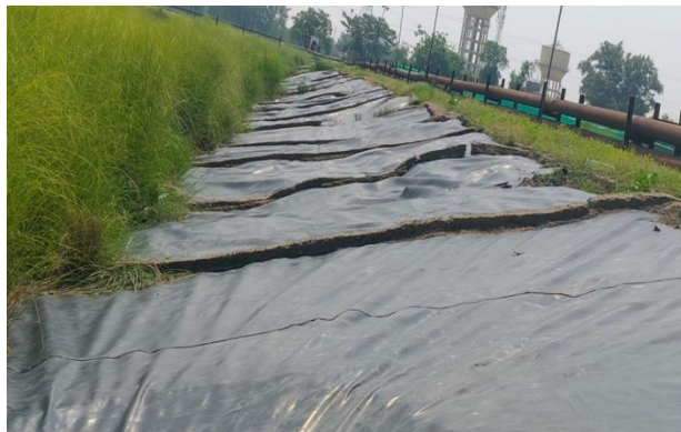
Laying of LDPE Sheet to mitigate dust emission slopes
