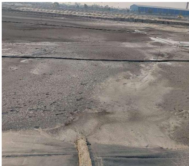
Wet Surface after Water Spray through Nozzles
