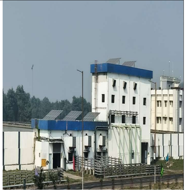
Roof top solar systems at reserve water
