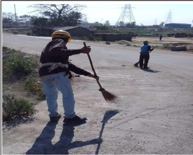
Removal of dust and Cleaning of Roads
