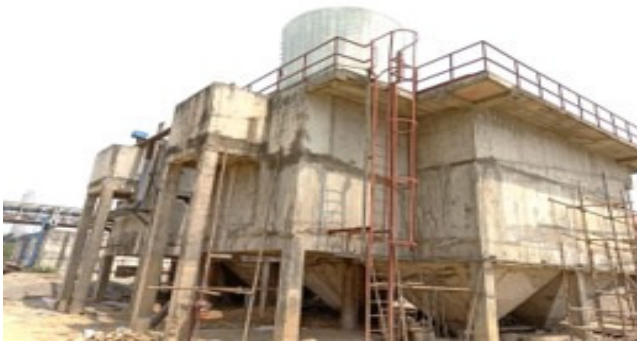
(Tube Settler and Neutralization Pit)
