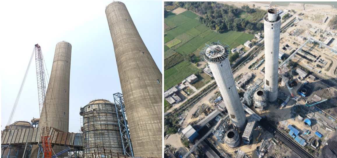
(Absorber and Chimney)
