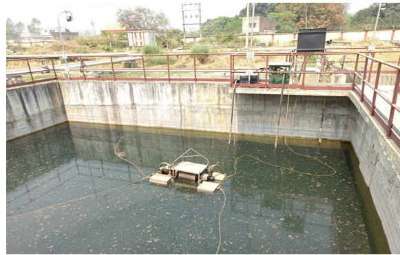
(Waste Service Water Sump with Oil Skimmer)
