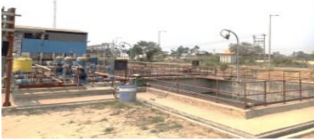
(Waste Service Water Sump with Oil Skimmer)
