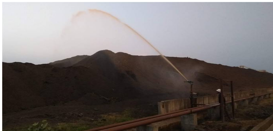
(Sprinkler at Coal Stack Yard)
