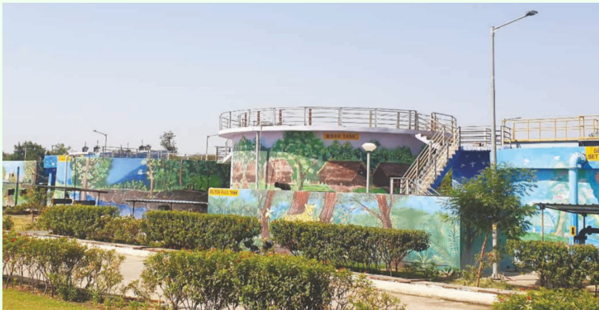
Sewage Treatment Plant
