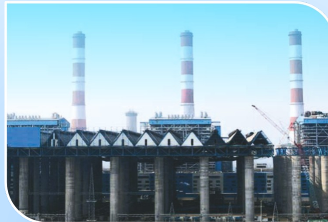
Air Cooled- Condenser at NTPC North-Karanpura
