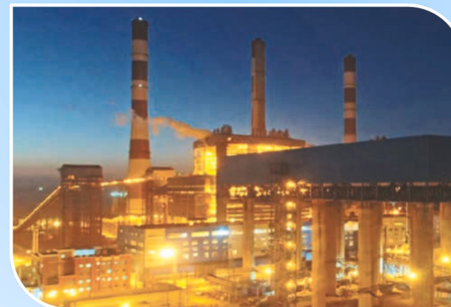
Air Cooled- Condenser at NTPC Patratu
