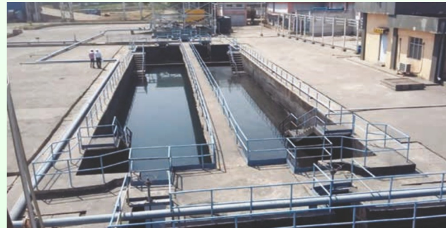
Coal Slurry Settling Pit
