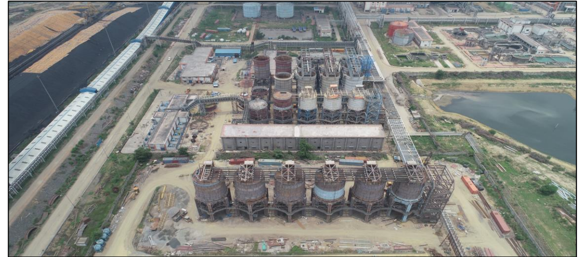
North-Karanpura has adopted the dry ash handling system
