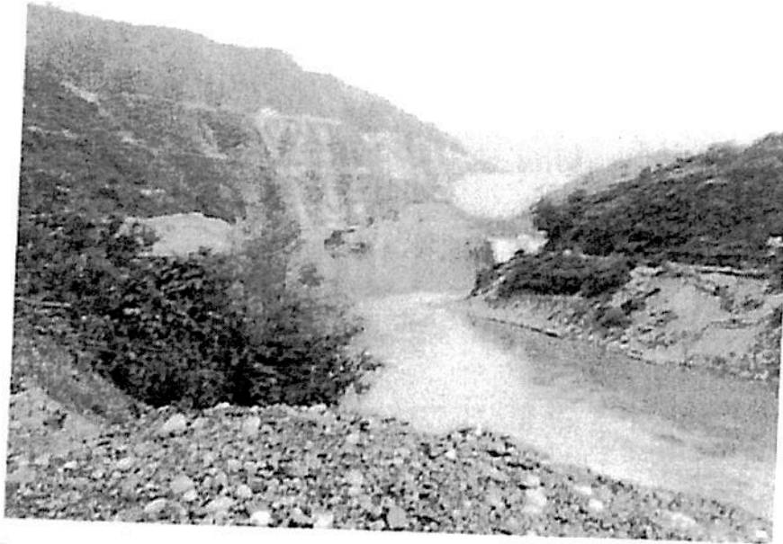
7. RHS of plunge pool, damaged needs protection.
