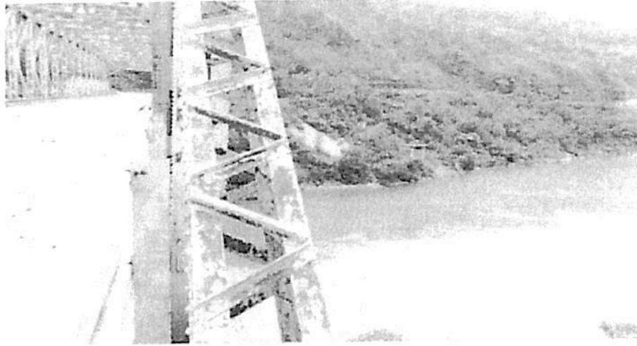
3. DS Maitri Setu Fully Protected: LHS River Satluj.
